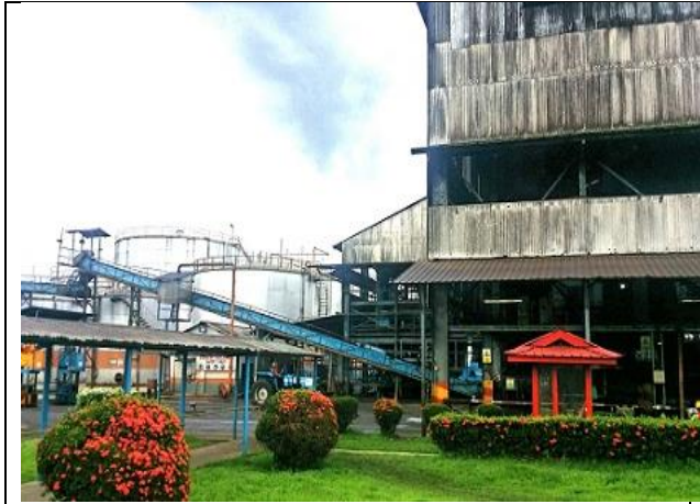
Pamol POM and CPO Storage tanks
